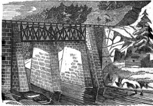
BRIDGE BELOW THE VIADUCT.
