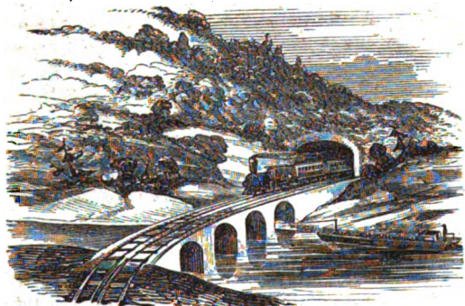
TUNNEL AND BRIDGE ABOVE PHOENIXVILLE.
