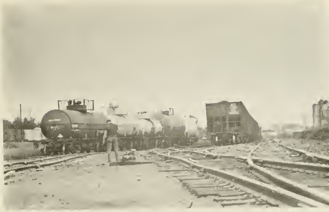
Switching tracks at Newberry Yard
