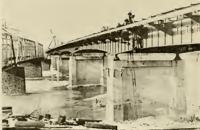
Former and present Market Street Bridges
