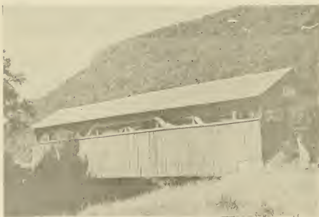
Covered bridge at Buttonwood
