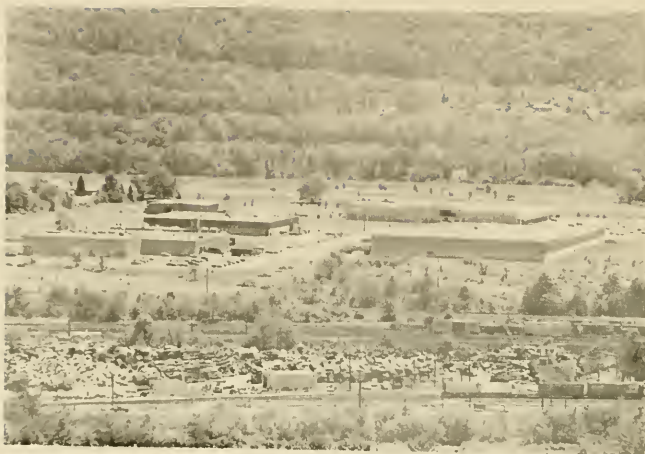
Williamsport Industrial Park
