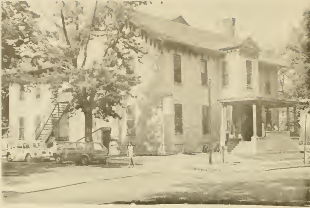
Bethune-Douglass Community Center (former Emery School)
