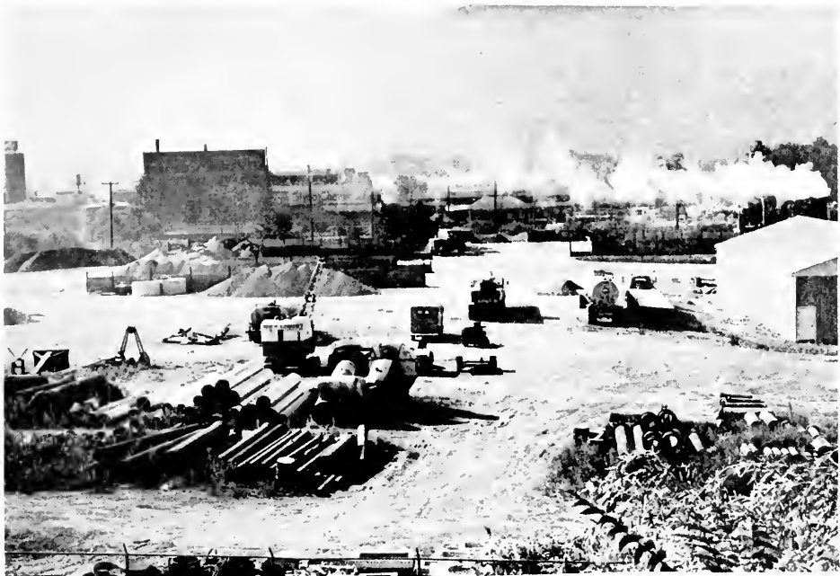
Glyco Chemical Company
