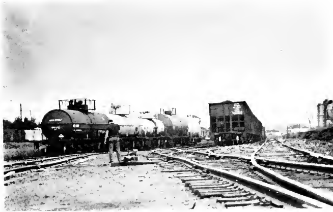
Switching tracks at Newberry Yard
