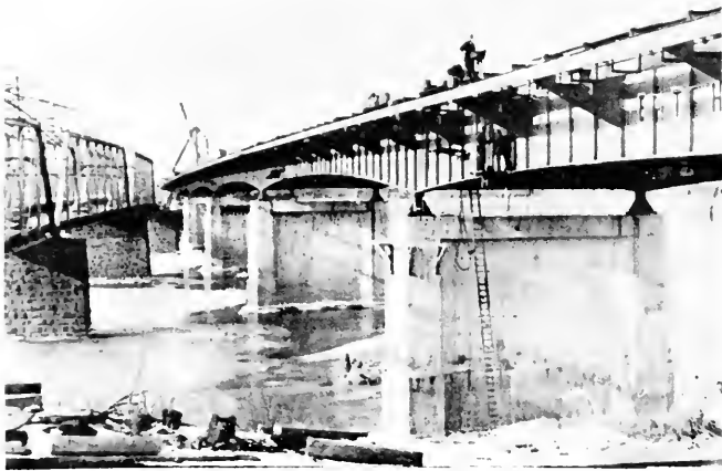
Former and present Market Street Bridges
