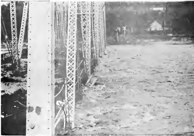
Memorial Avenue Bridge, Williamsport, during Agnes flood
