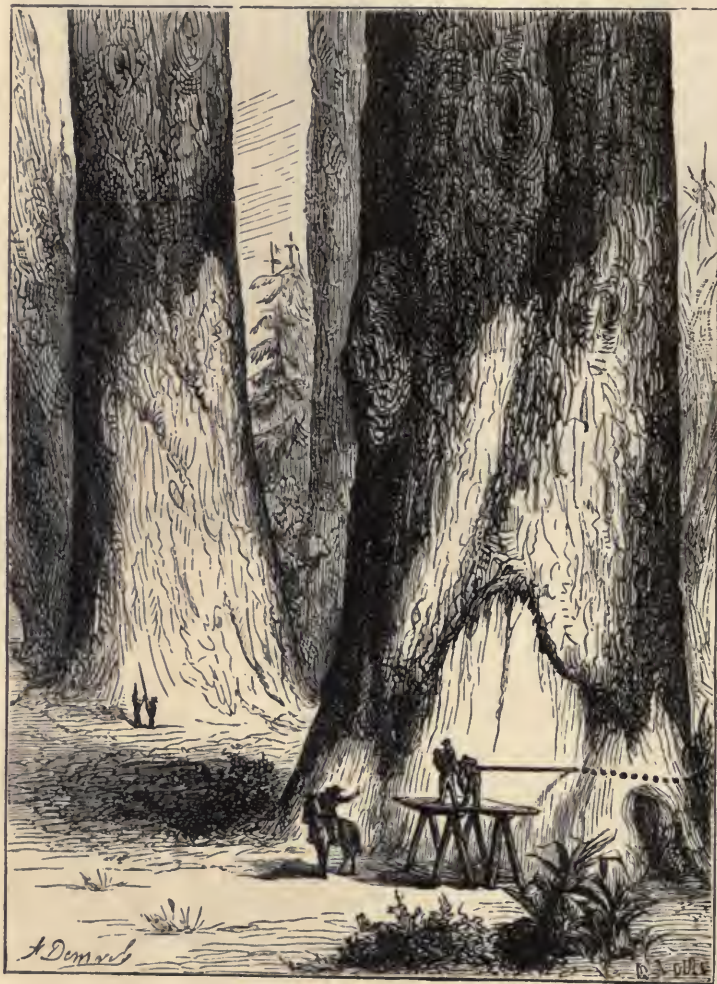
PREPARING TO FELL BIG TREE.
