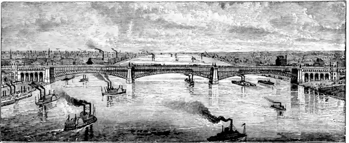
GREAT STEEL BRIDGE AT ST. LOUIS, CROSSING THE MISSISSIPPI.*
