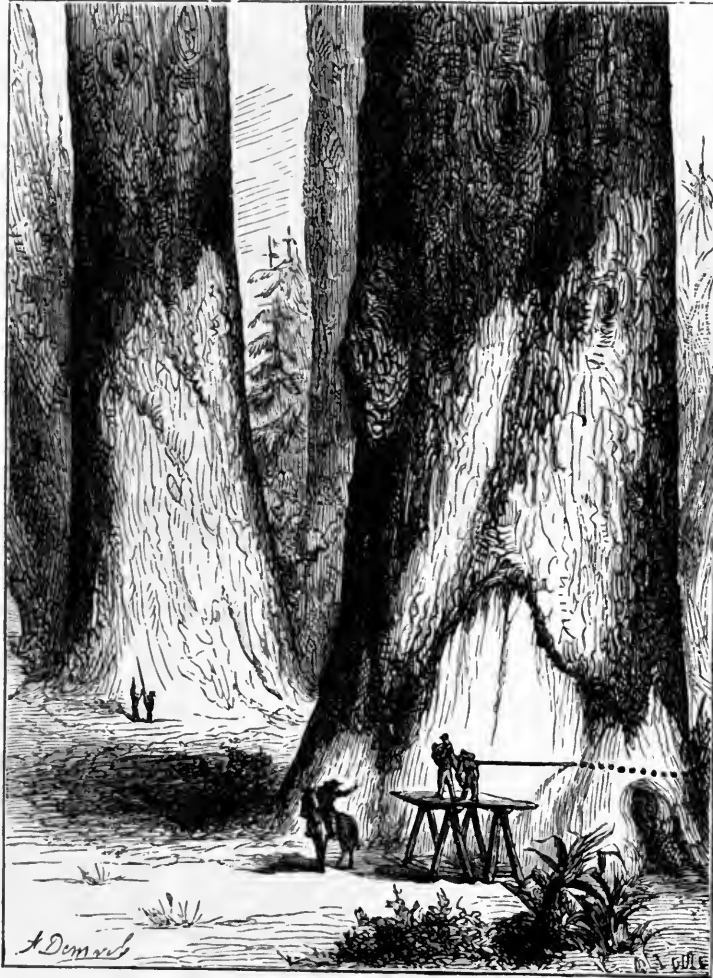
PREPARING TO FELL BIG TREE.
