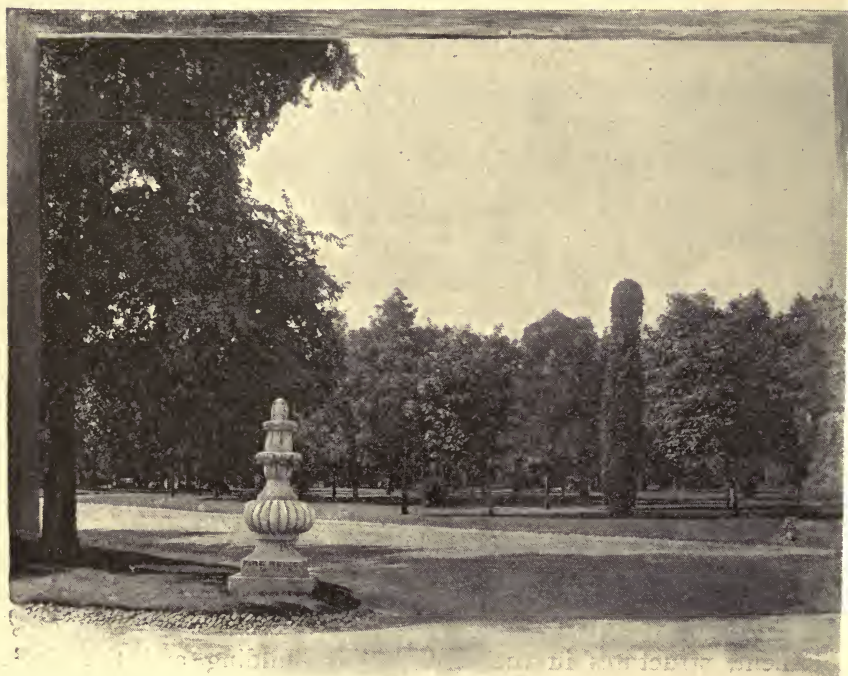
RELIC OF OLD COURT-HOUSE AFTER THE FIRE.
