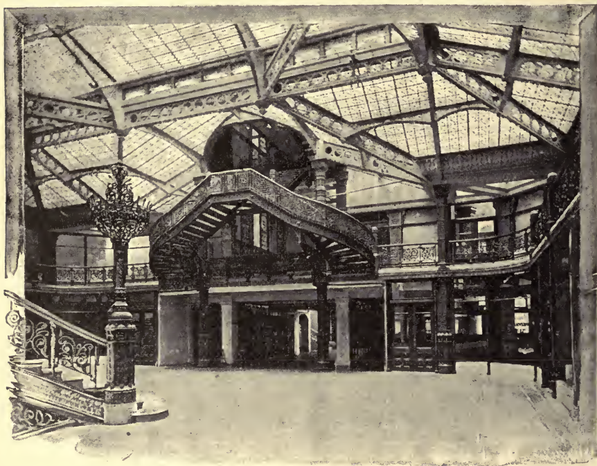
INTERIOR OF PRESENT ROOKERY BUILDING.
