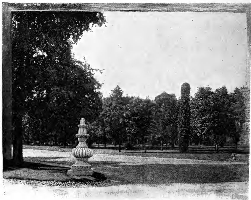
RELIC OF OLD COURT-HOUSE AFTER THE FIRE.
