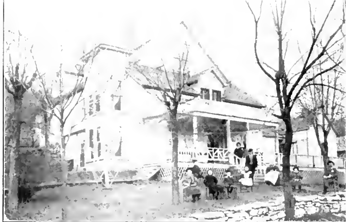
RESIDENCE AND HOTEL OF R. CALDWELL
