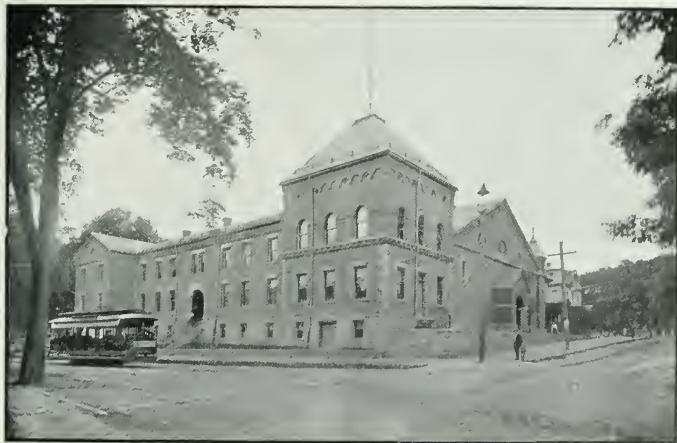
THE ARMORY—COIT AND WASHINGTON STREETS.
