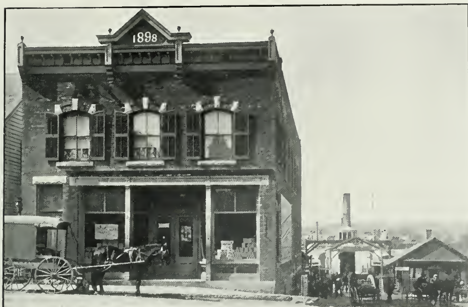
FERRY LANDING AND ALLYN BLOCK—GROTON.
