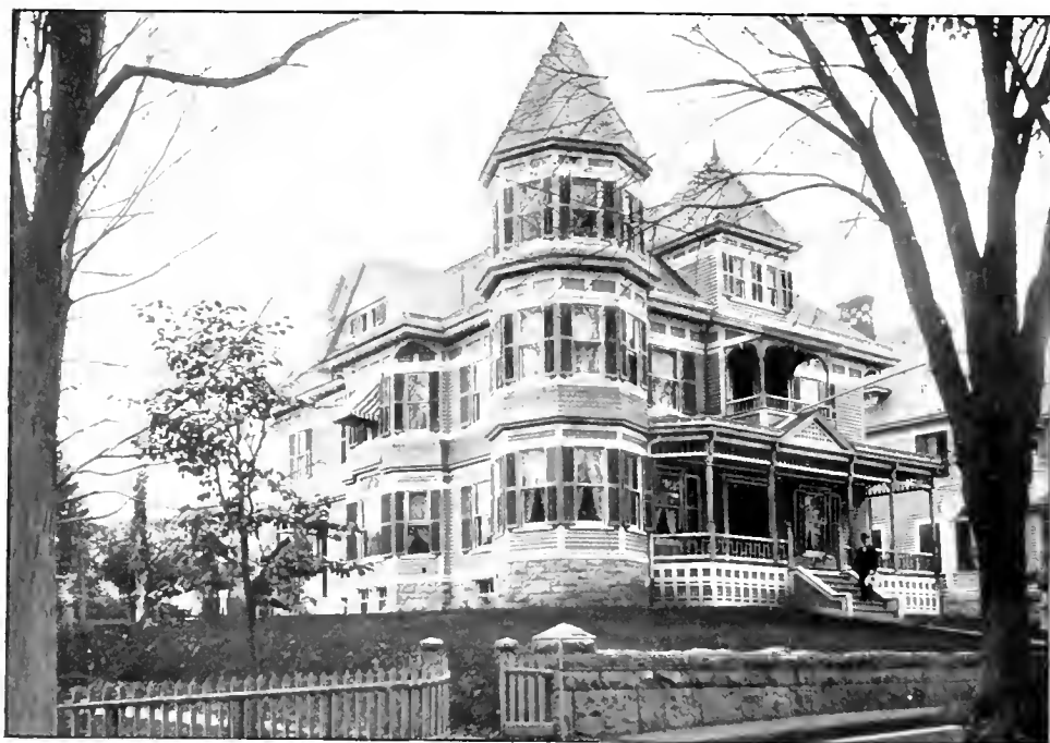
RESIDENCE OF MORRIS W. BACON — 2 CHANNING STREET.
