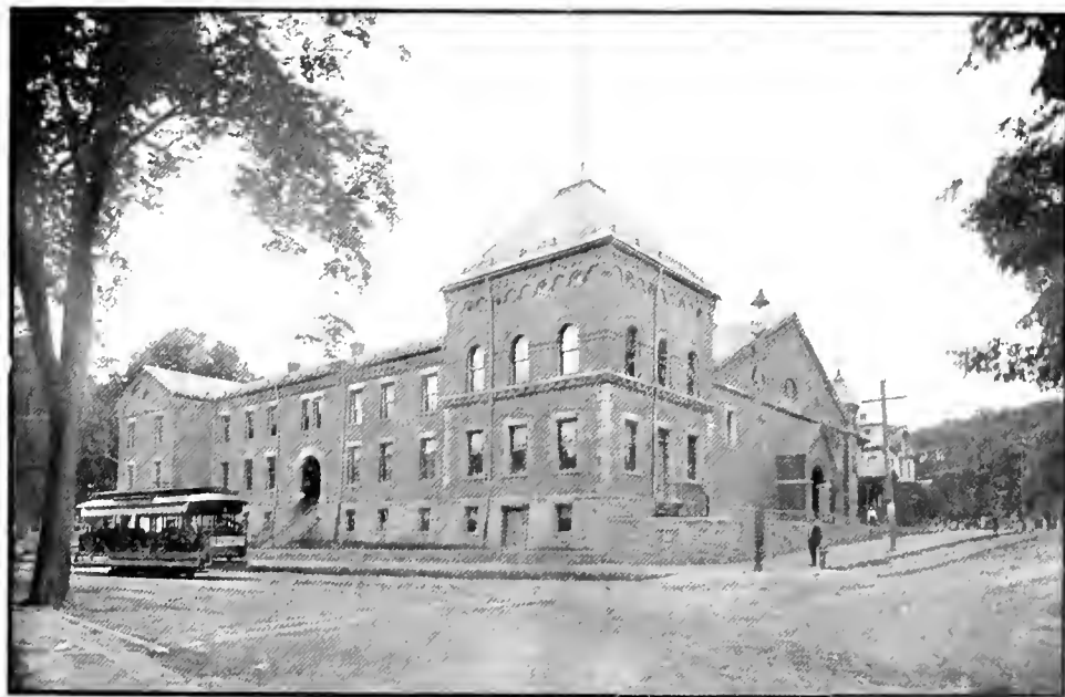
THE ARMORY—COIT AND WASHINGTON STREETS.
