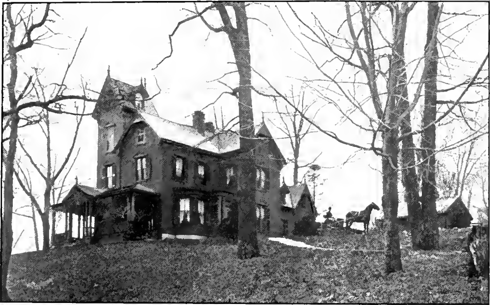
RESIDENCE OF HENRY C. JOHNSON, PRESIDENT OF THE WILLIAM G. JOHNSON COMPANY—MONTVILLE, CONNECTICUT.
