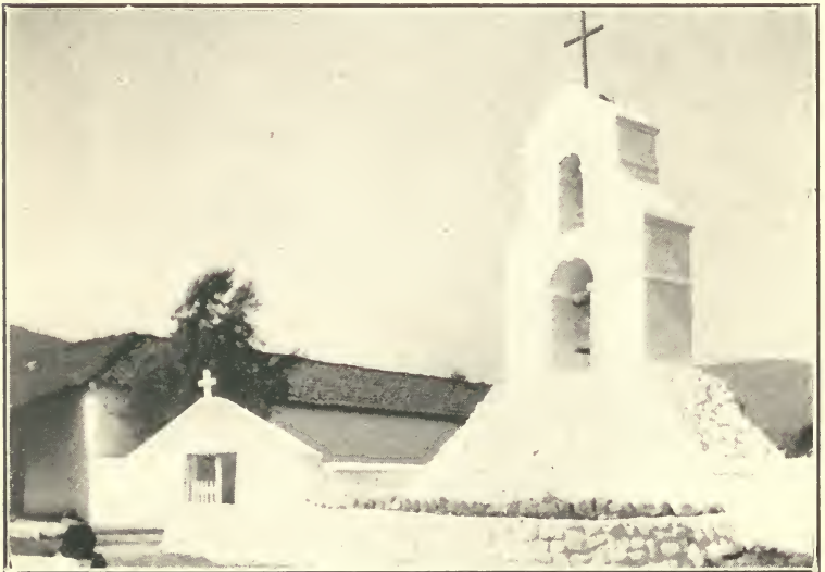
The Pala Bell Tower After Rebuilding.
