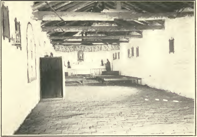
The Interior of Pala Chapel After the Restoration.
