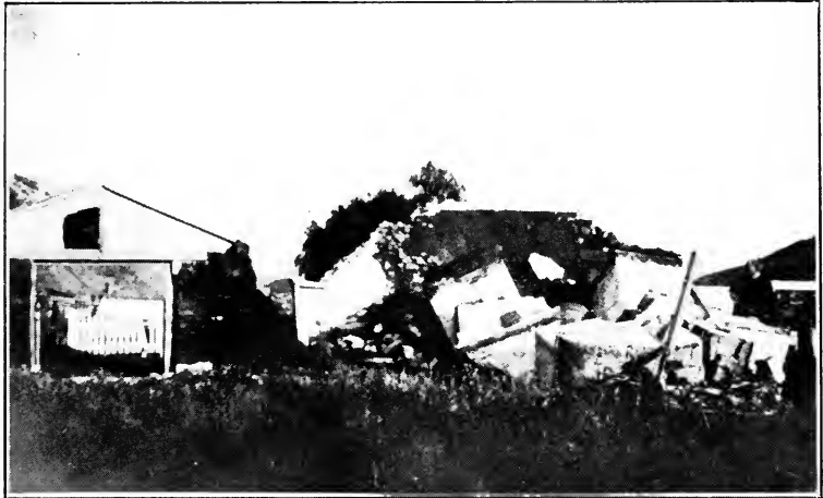
The Ruins of the Pala Campanile, After Its Fall in January, 1916.
