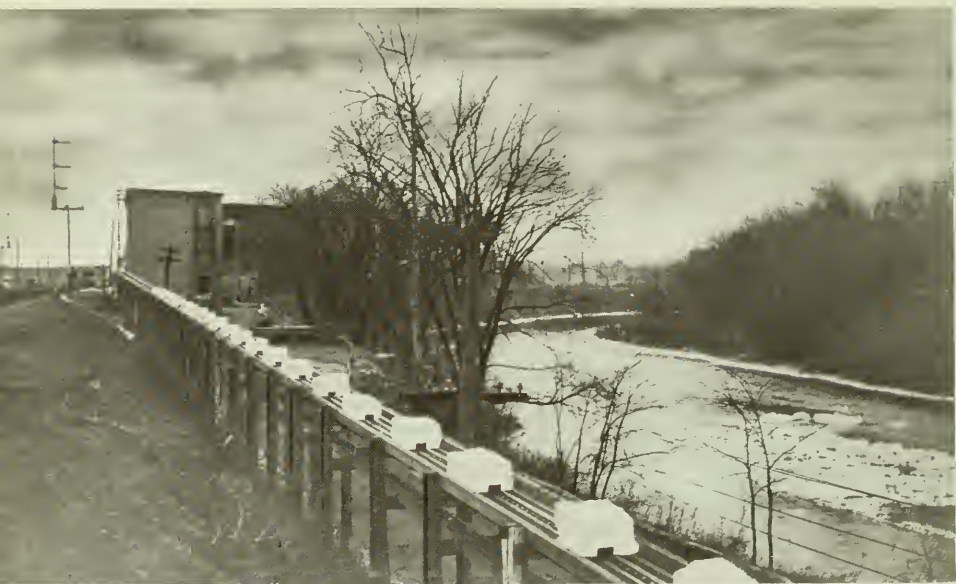
HYGIENIC ICE ON THE RUNWAY, TO STORAGE HOUSE OF THE RAMAPOGUE ICE COMPANY, WEST SPRINGFIELD.
