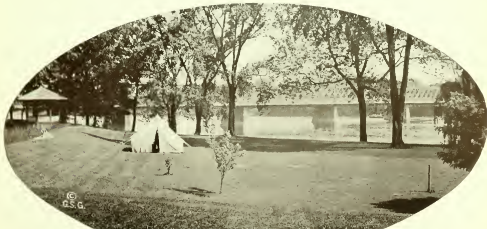
NORTH END BRIDGE OVER THE CONNECTICUT RIVER FROM GROUNDS OF FRANK L. WORTHY.
