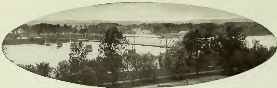
VIEW OF SOUTH END BRIDGE looking from Long Hill, Springfield, to Agawam, where the Agawam River comes into the Connecticut. If the River Front Plan, now being considered by the City Government is carried out, the N. Y., N. H. & H. R. R. will cross the Connecticut River below this bridge and have its freight terminal on the West Springfield meadows, adjoining the N. Y. Central yards, thus doing away with the present tracks on Springfield's river front.
