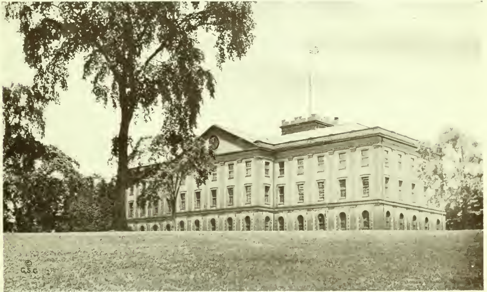
MAIN ARSENAL, UNITED STATES ARMORY GROUNDS.
