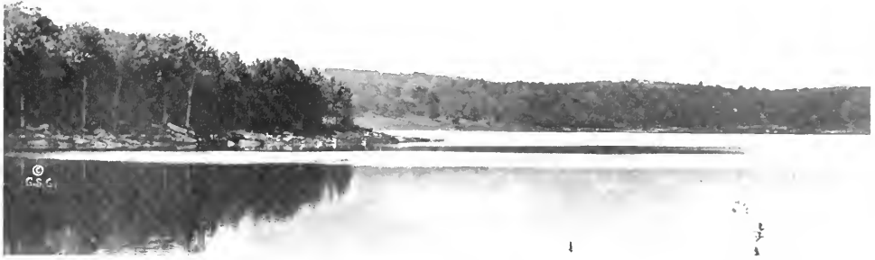
BORDEN BROOK RESERVOIR which has a capacity for storing eighteen months' supply of water.
