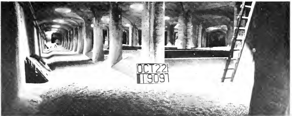
INSIDE THE FILTRATION BEDS BEFORE THE WATER WAS LET IN.
