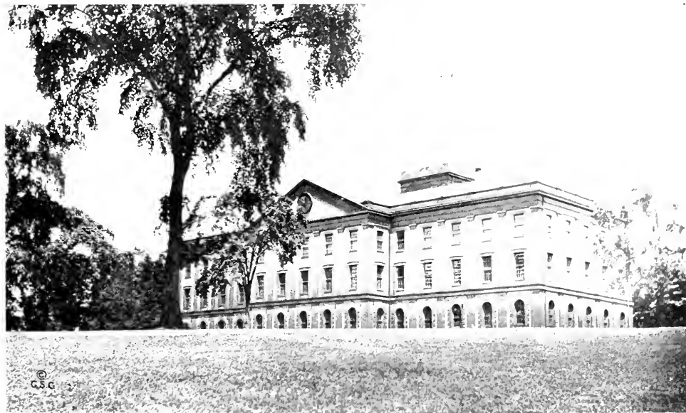
MAIN ARSENAL, UNITED STATES ARMORY GROUNDS.
