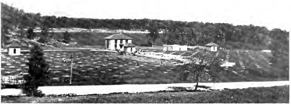
SPRINGFIELD'S MODERN FILTRATION BEDS WHERE LITTLE RIVER WATER IS MADE ABSOLUTELY PURE.
