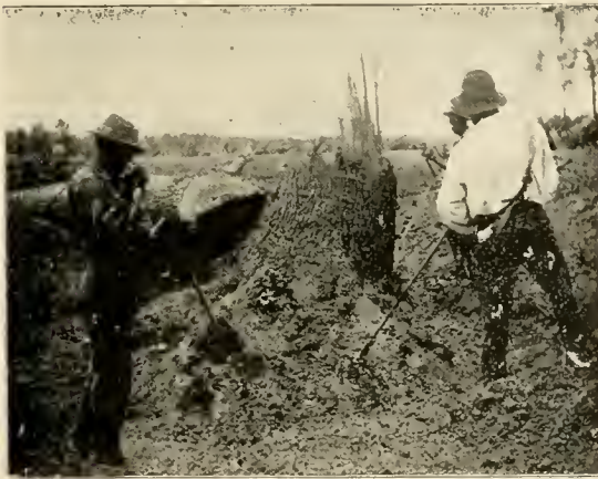
DRILLING FOR A BLAST.
