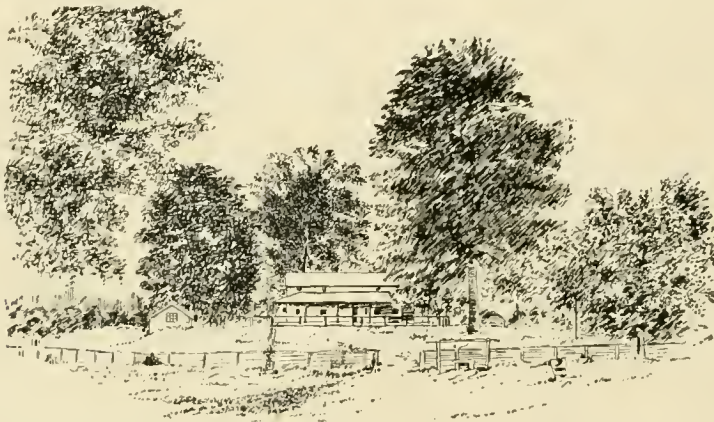
A PLANTER'S HOME, BUILT ON AN INDIAN MOUND.
