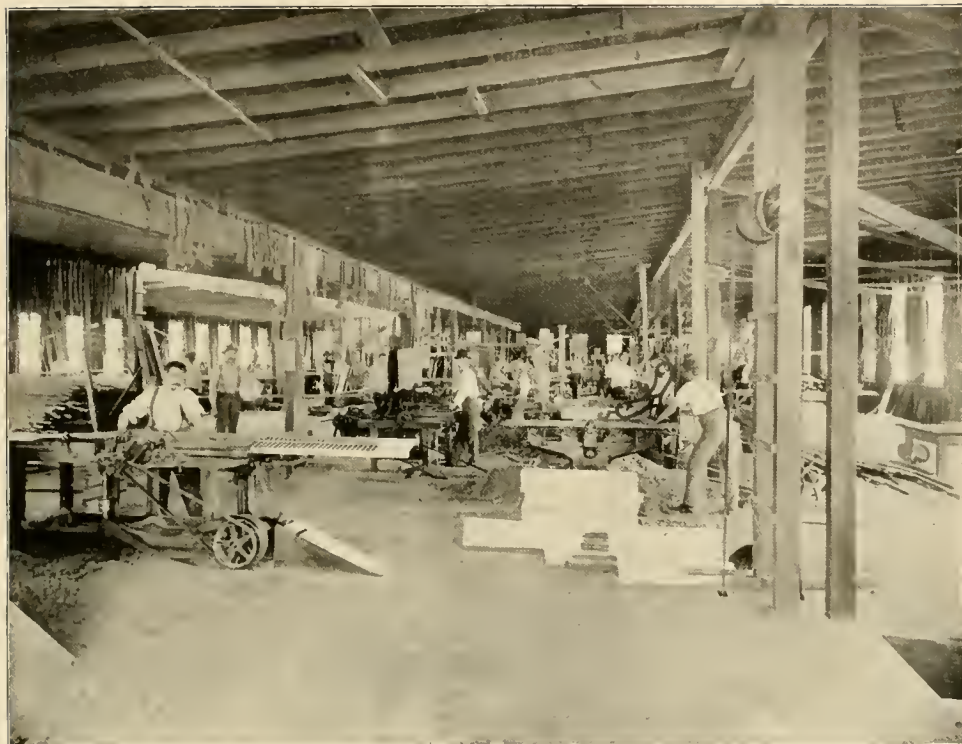
INTERIOR OF WORKSHOP.
