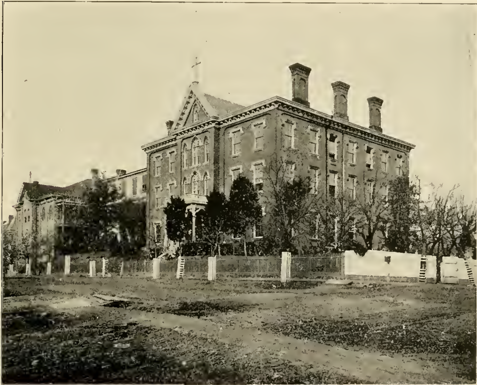
VIEW OF ST. FRANCIS XAVIER ACADEMY FROM CRAWFORD STREET.
