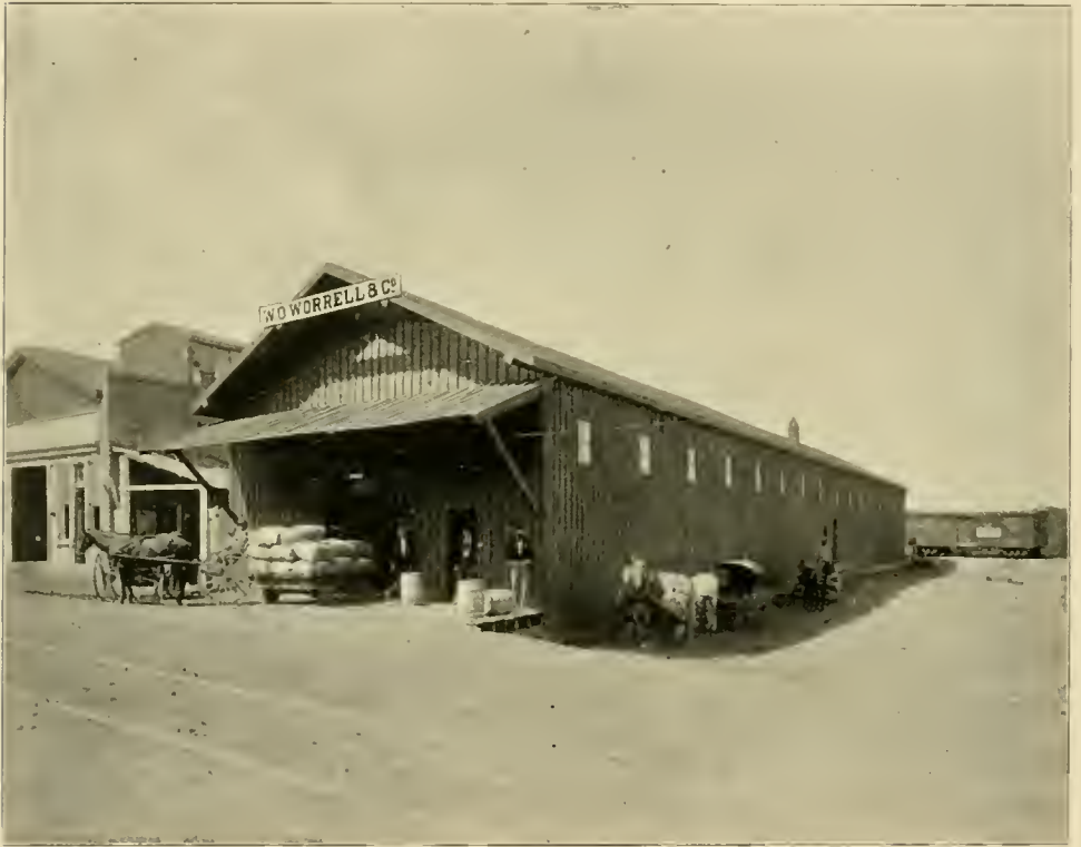
VIEW OF WAREHOUSE FROM THE Y. & M. V. RAILROAD TRACKS.
