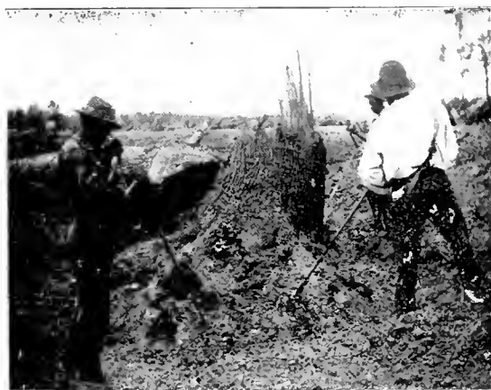
DRILLING FOR A BLAST.
