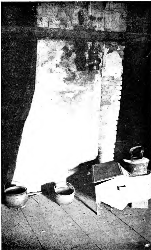
THE ATTIC CHIMNEY
