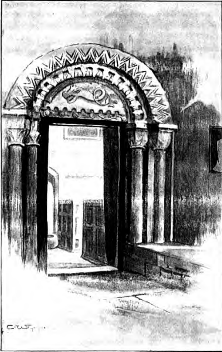
SOUTH DOORWAY, AUSTERFIELD CHURCH.
