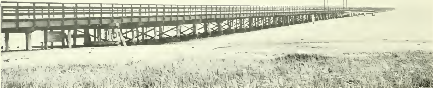
POWDER POINT BRIDGE, DUXBURY
