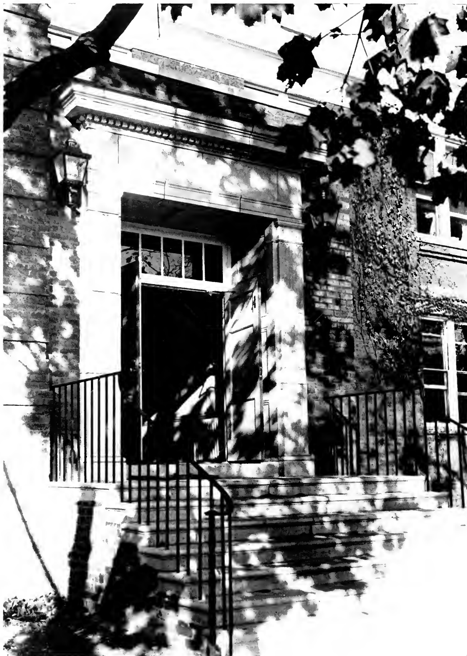
Remodeled Entrance to North Spencer
