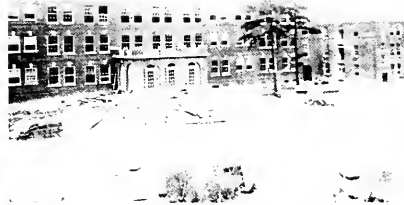
QUADRANGLE UNDER CONSTRUCTION 1912
