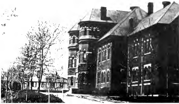
EARLY VIEW OF THE ADMINISTRATION BUILDING
