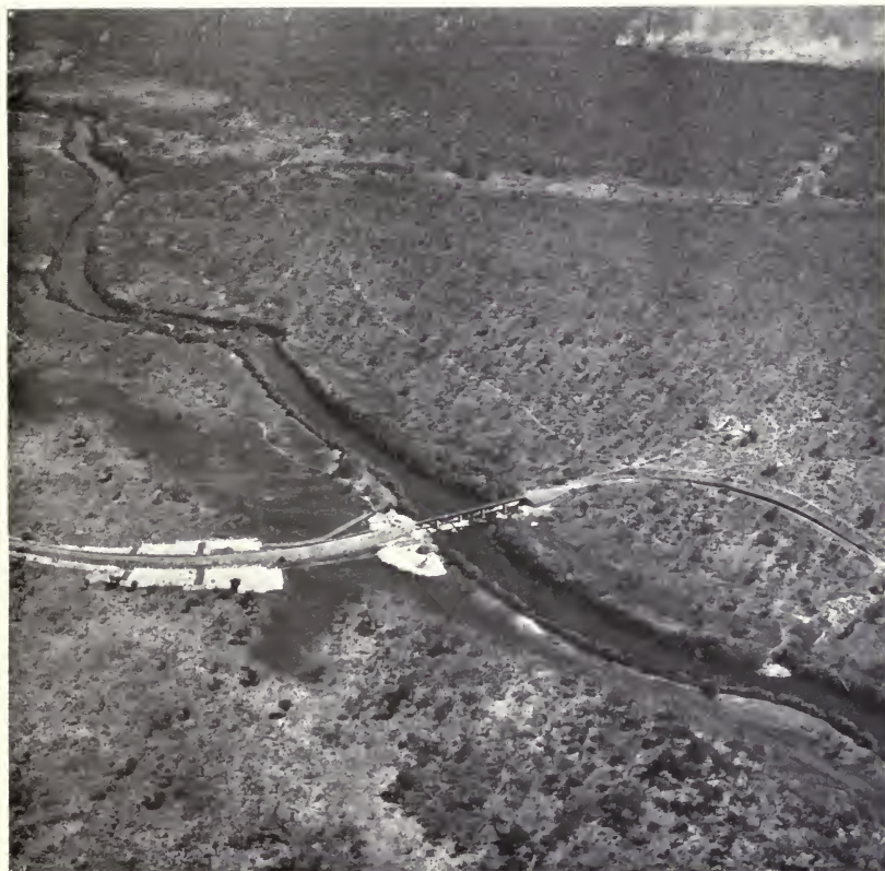
FIG. 172—Nkana Railway Bridge over Kafue River, Northern Rhodesia. Railroad extension opened in the summer of 1930. Smoke from bush fire in background. (Aircraft Operating Co., London.)
