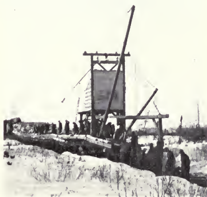
FIG. 120—Men laying steel at a mile a day during below-zero weather on the Churchill extension, Hudson Bay Railway. (Canadian National Railways.)
