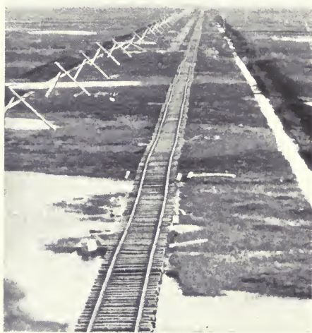
FIG. 3—Telephone line on temporary tripods and new track in undeveloped country, Hudson Bay Railway. (Canadian National Railways.)
