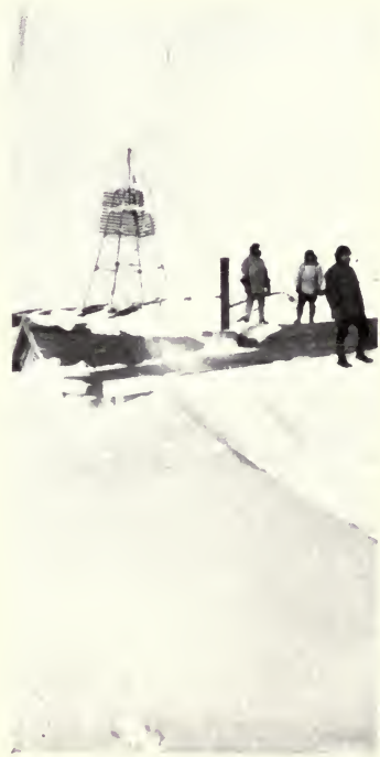
FIG. 48—Wireless station, Churchill, Manitoba. (Nat. Resources Intell. Service, Dept. of the Interior, Canada.)
