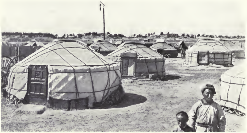
FIG. 197—Mongolian habitations. The farms are built of kaoliang stalks and covered with felt. (South Manchuria Railway Co.)
