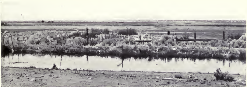
FIG. 66—Southeastern corner of reclaimed portion of Tule Lake floor, California, looking west.
