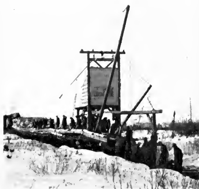
FIG. 120—Men laying steel at a mile a day during below-zero weather on the Churchill extension, Hudson Bay Railway. (Canadian National Railways.)
