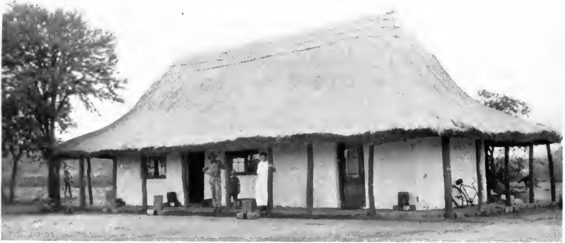
FIG. 162—Settler's home, second stage, Southern Rhodesia. (Photograph by G. W. Marshall; courtesy High Commissioner for Southern Rhodesia, London.)
