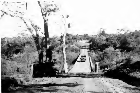
FIG. 165—Road improvement in Southern Rhodesia: low-level bridge over a stream. (High Commissioner for Southern Rhodesia, London.)
