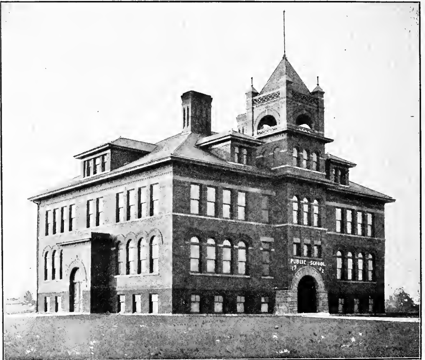
PUBLIC SCHOOL BUILDING, POCAHONTAS, 1902.
