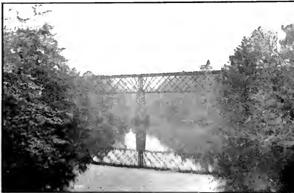
R. W. & O. Railroad Bridge.
