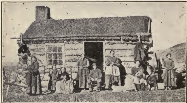
Pioneer cottage. Several families working together.
