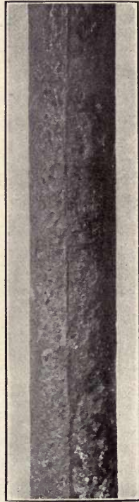
Cast Iron Pipe 100 Years Old, From Godesberg, Germany
