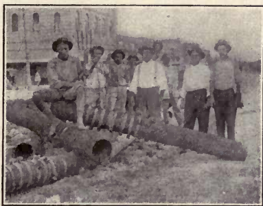
Wood Pipe Replaced With Cast Iron Pipe at Rogers Texas
