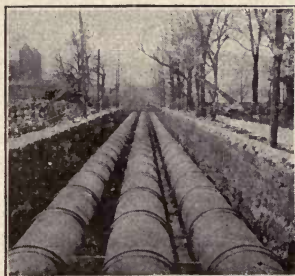
Three Lines of 60-Inch Cast Iron Pipe
