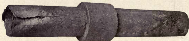
Fig. 7—Wrought Iron and Cast Iron Pipe Coupled Together for Service to Compare Durability
