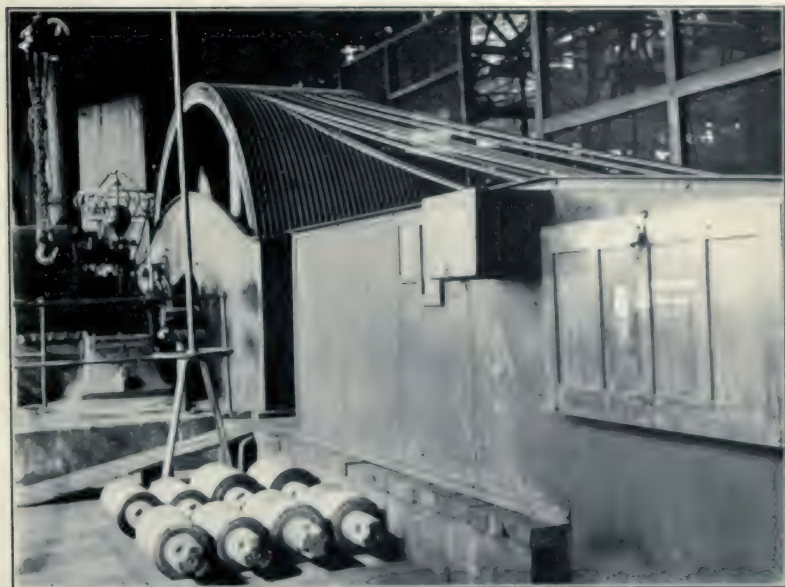
PLATE 5.—VIEW OF ROPE DRIVE FOR ROD MILL, SHOWING STEEL PLATE ENCLOSURE
