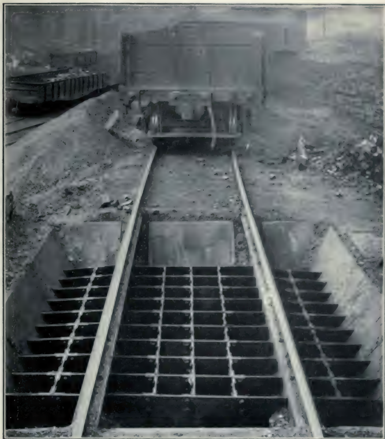
PLATE 18.—GRILL WORK PROTECTION FOR BINS AND HOPPERS Sometimes a workman falls through a car of coal or ore, into the bin underneath the track, where he is liable to be suffocated if not gotten out promptly
