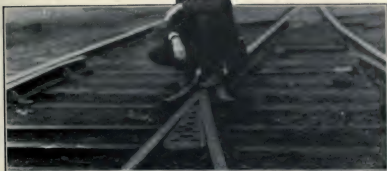
PLATE 17.—GUARD FOR FROGS MADE OF STEEL PLATE
