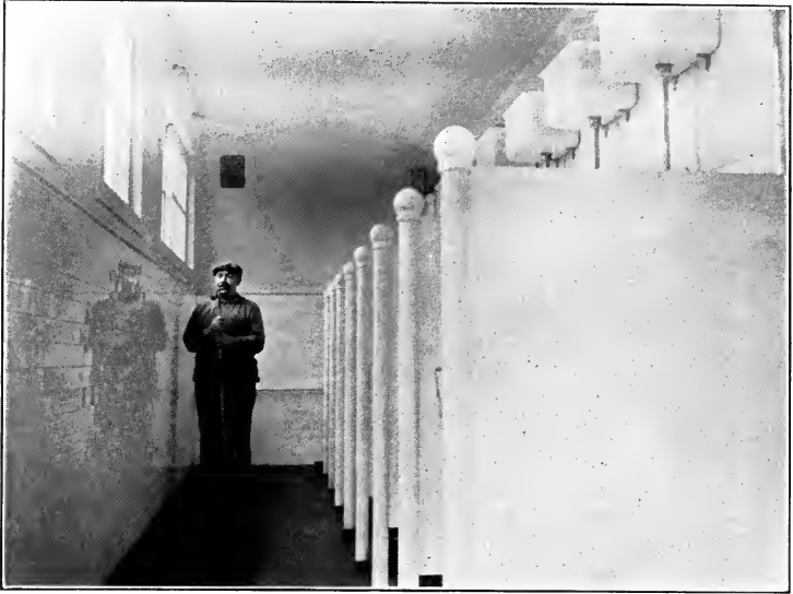
CLOSETS IN COMFORT BUILDING AT LUCY FURNACE
