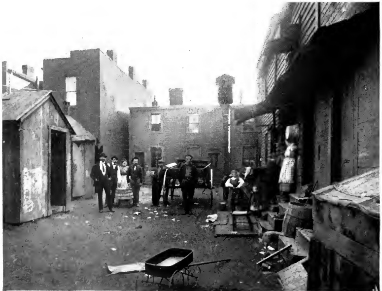
HAZEL ALLEY, MCKEESPORT Vaults and living rooms in close proximity
