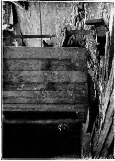
HYDRANT ADJACENT TO VAULT The only water supply for nine families
