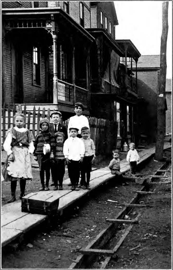
MILLER STREET, DUQUESNE Open drain at side of street
