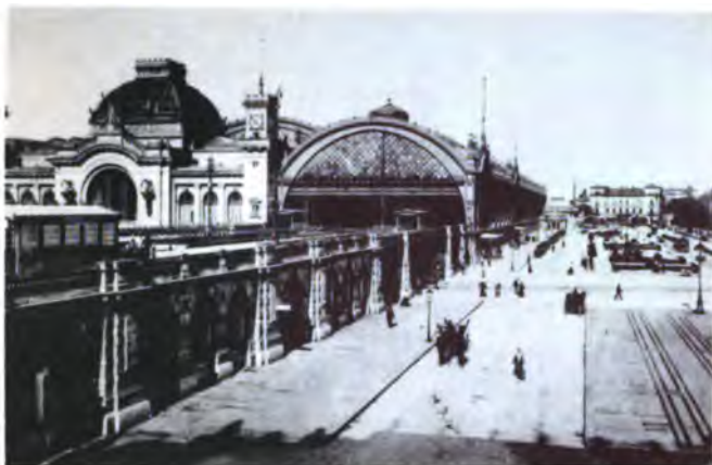
LXXVI. DRESDEN. VIADUCT AND RAILWAY STATION (HAUPT BAHN-HOF) PASSING ABOVE THE NORMAL STREET LEVEL, ILLUSTRATING THE TYPE PROPOSED IN THE OVERHEAD SCHEME FOR RAILWAY STATIONS WEST OF THE RIVER.
