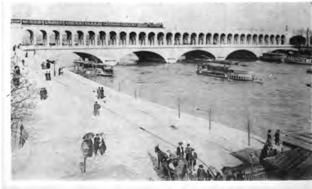
LXXXIII. THE VIADUCT AT AUTEUIL OVER THE RIVER SEINE, PARIS, FRANCE.
