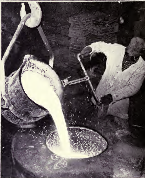
Cooper Alloy Foundry worker pours metal into spinning mold to produce high standard castings required in turbojet plane components.
