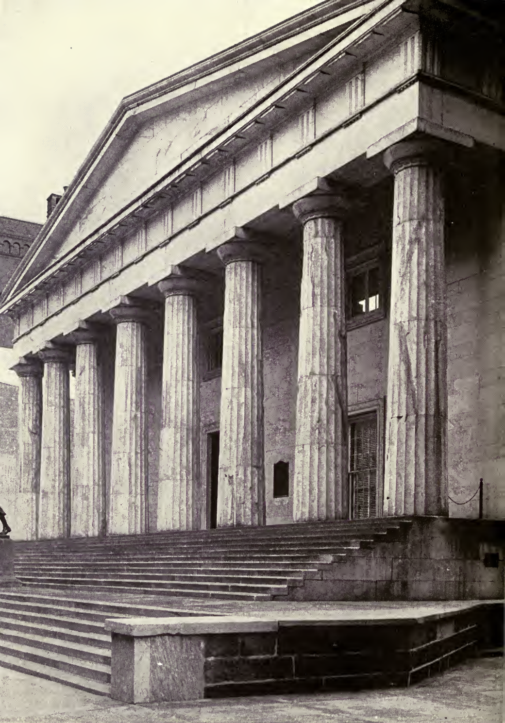
The Old Philadelphia Custom House National Historic Site, Philadelphia, is a notable example of Greek Revival Architecture in America. It was built as the Second Bank of the United States and was the center of the famous Andrew Jackson-Nicholas Biddle political battle over the rechartering of that institution.
