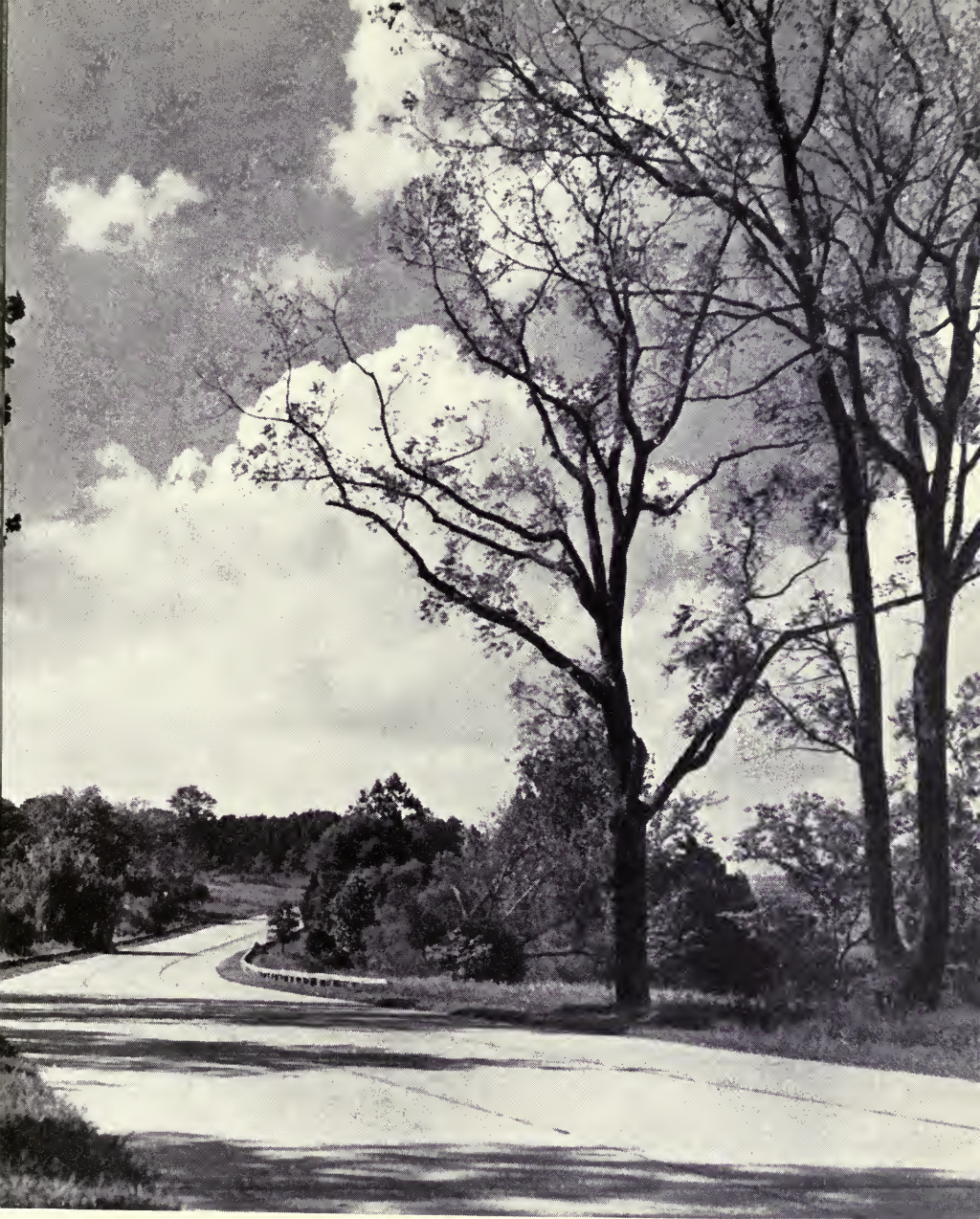
Views of Colonial Parkway along the York River. This section has been complete for several seasons.
