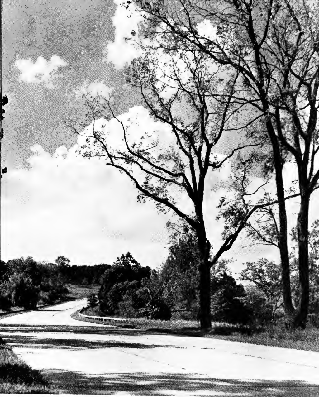
Views of Colonial Parkway along the York River. This section has been complete for several seasons.
