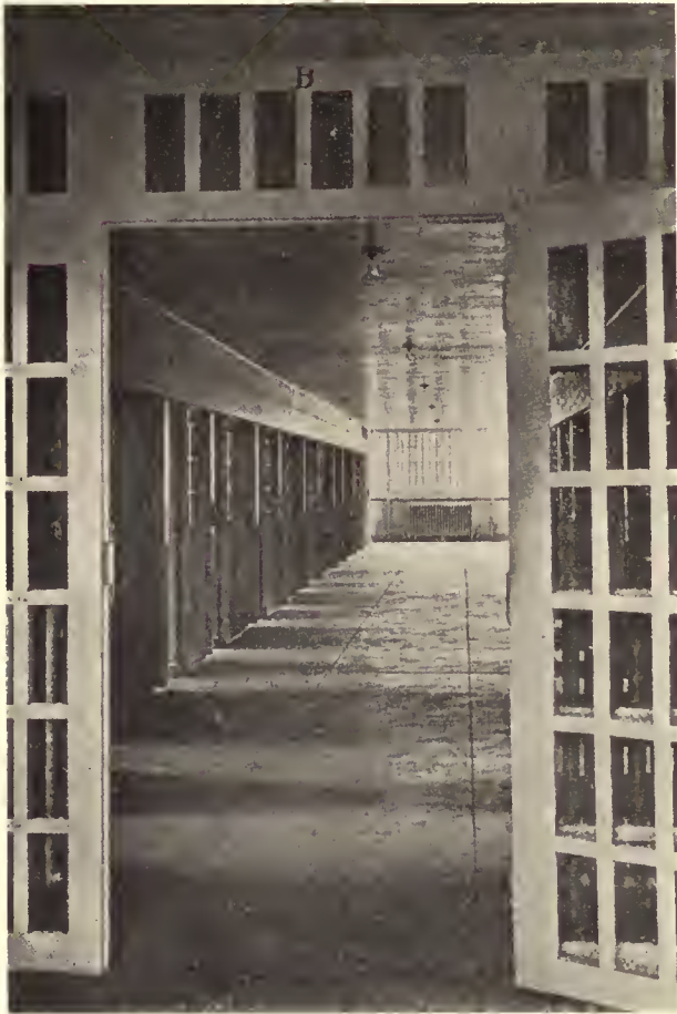
CELL BLOCK CORRIDOR
