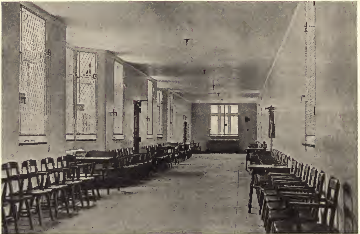
RECREATION CORRIDOR LOOKING TOWARD CELL BLOCK
