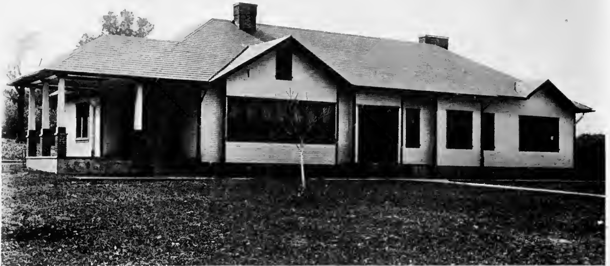
THORN HILL SCHOOL, WARRENDALE, PENN.—ONE-STORY COTTAGE Designed by FRANKLIN H. BRIGGS, Superintendent
