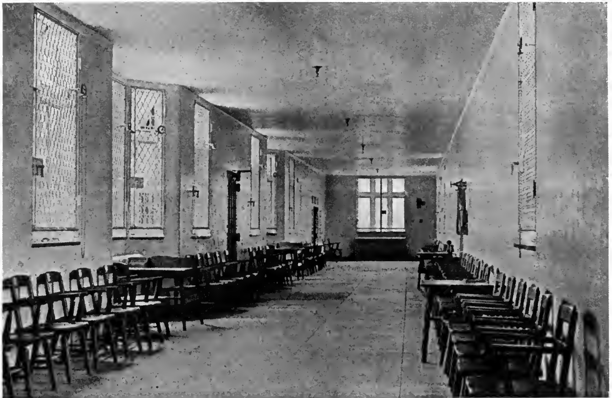
RECREATION CORRIDOR LOOKING TOWARD CELL BLOCK
