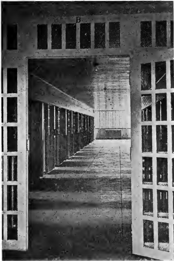
CELL BLOCK CORRIDOR
