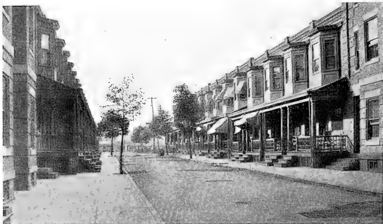
Fig 3. A residence street insufficiently shaded. See Figs. 4 and 26.
