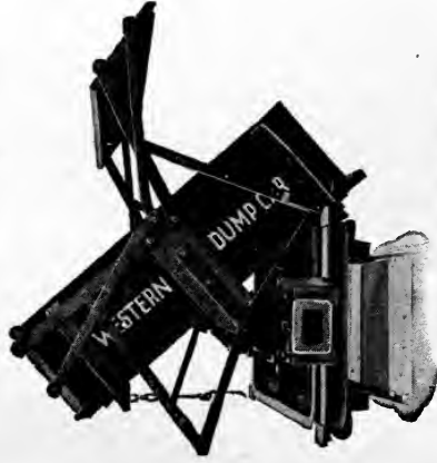
1½-yd. Car in Dumped Position
