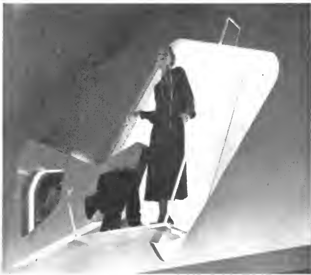
The Solar Plastic Products Company, Brooklyn, New York, fabricated this item for the new Bond Store at 35th Street and Fifth Avenue, New York City. It was designed by Morris Lapidus, architect.
