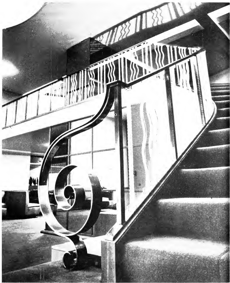
Plastics used for interior decoration on stair railing. (Courtesy Modern Plastics)
