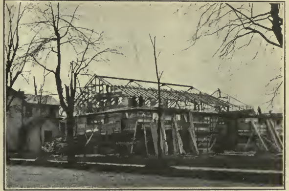
IT BEGINS TO LOOK LIKE A BUILDING
