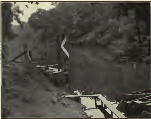
CANOE LANDING AND SWIMMING PIER Slippery Rock State Normal School
