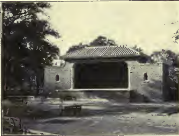
LITTLE THEATRE, FT. WORTH, TEXAS Combined Shelter House and Comfort Station
