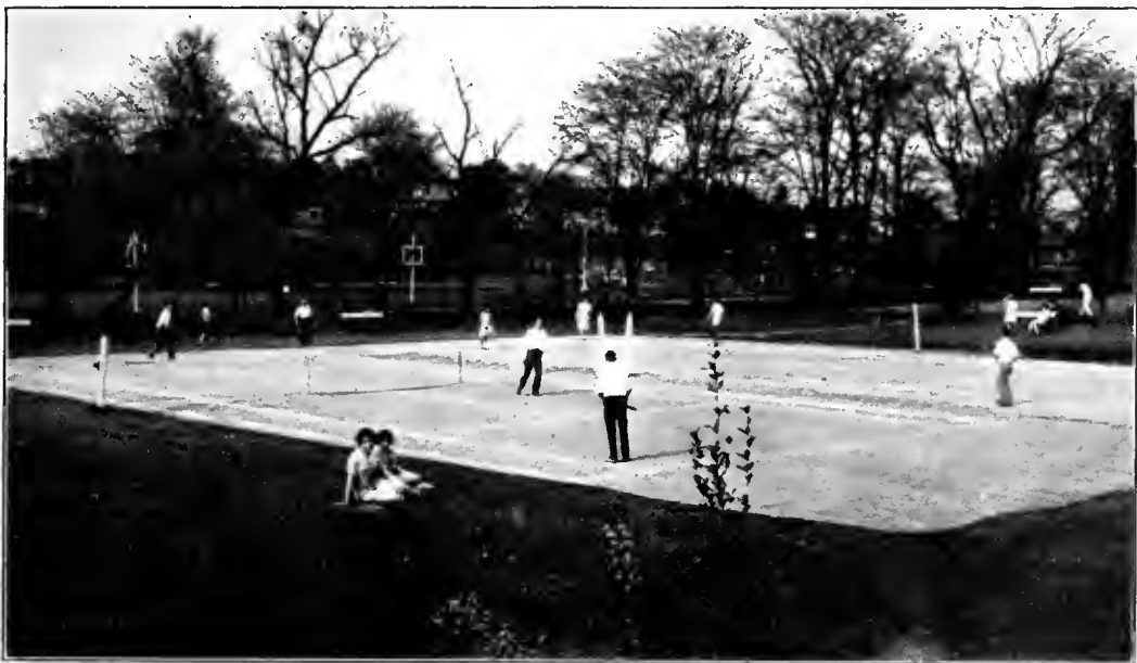
THE TENNIS COURT, HARMON PARK, LEBANON, OHIO
