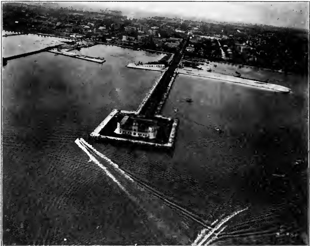
RECREATION PIER, ST. PETERSBURG, FLA.
