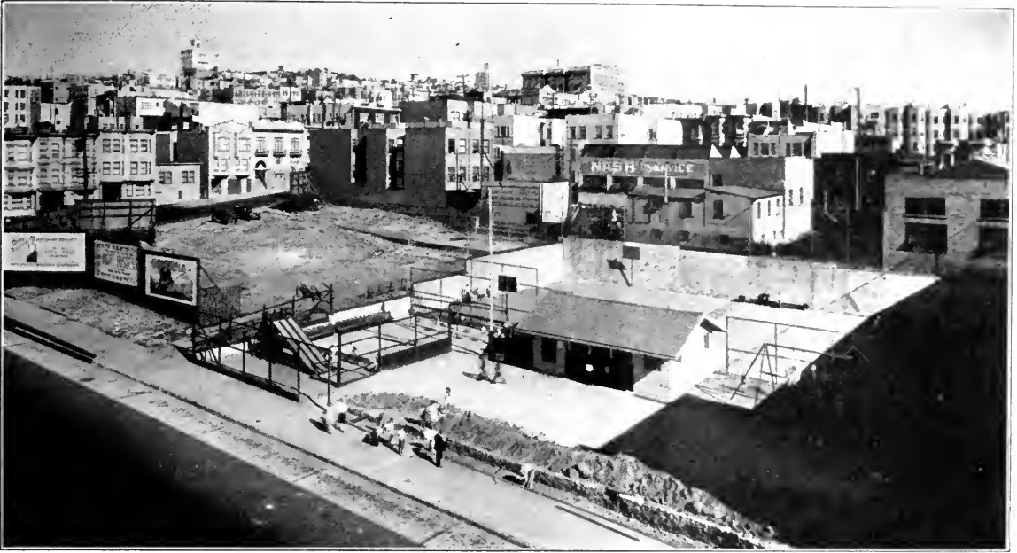
THE HELEN WILLS PLAYGROUND, SAN FRANCISCO, BEFORE RECONSTRUCTION
