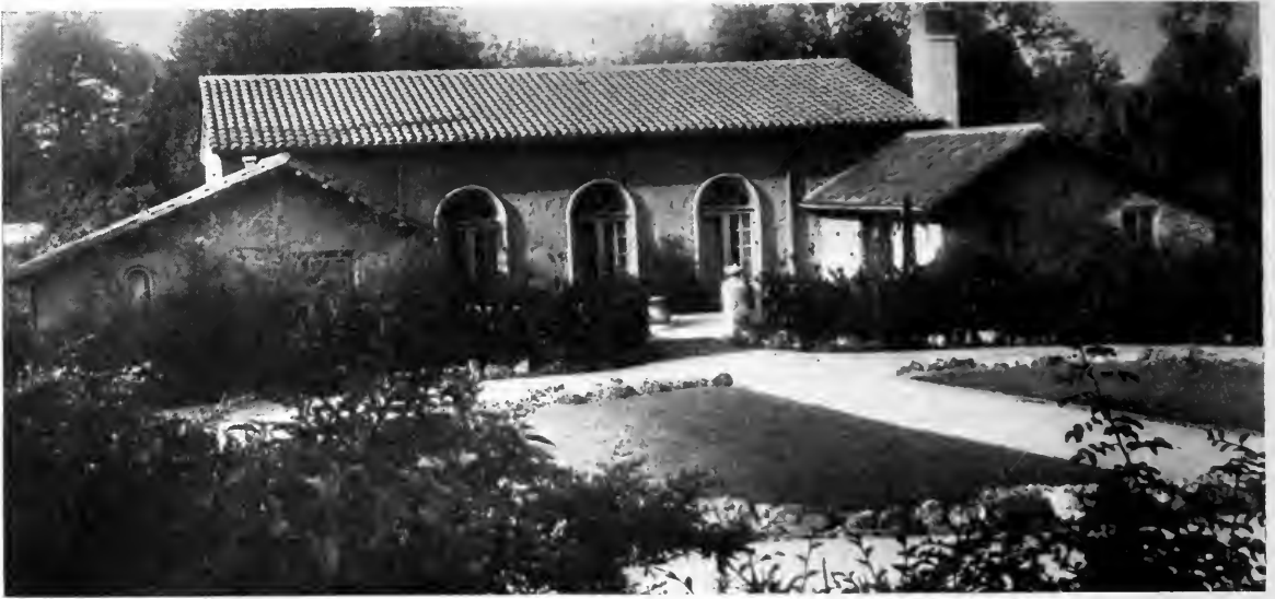
Piedmont's Community Recreation Center
