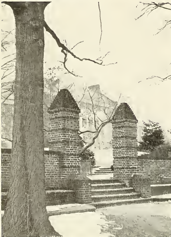
Stone walls by the walkways.
