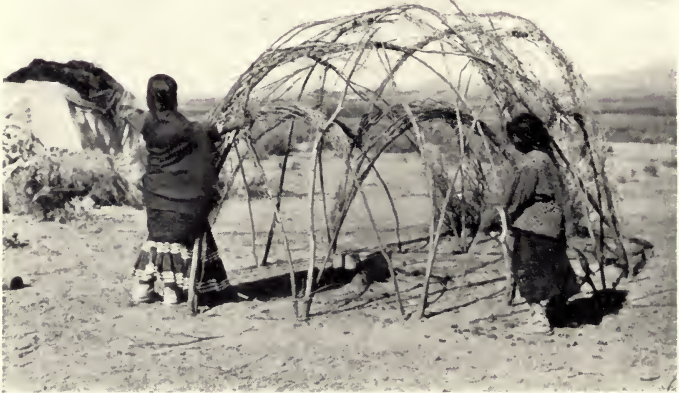
San Carlos Apache Women Building a House.
