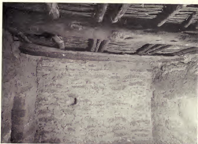
Roof. Spruce Tree Ruin. (Photo by Nusbaum.)
