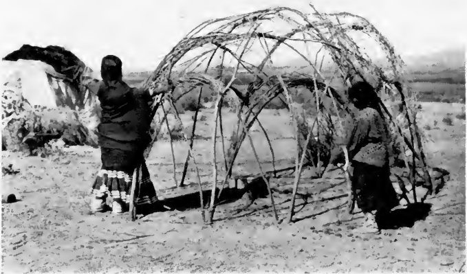
San Carlos Apache Women Building a House.
