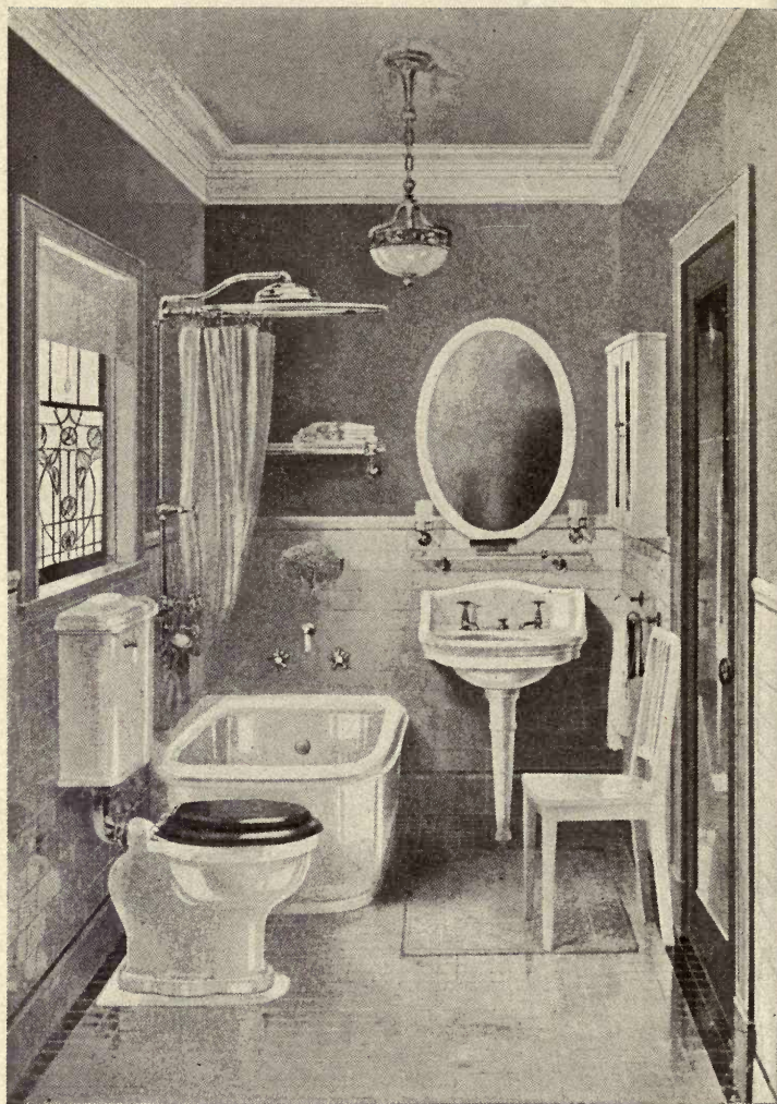
MODERN BATHROOM SHOWING EXCELLENT ARRANGEMENT OF FIXTURES IN SMALL SPACE
