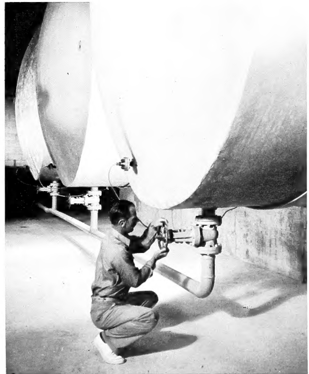
Laboratory sewage is heated in these 30,000-gallon tanks for decontamination.
