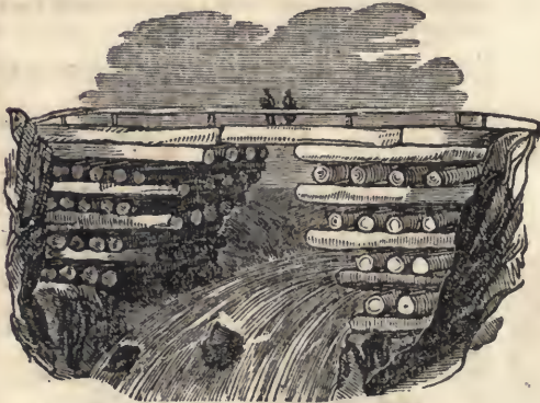
Bridge and Mountain torrent in Norway.
