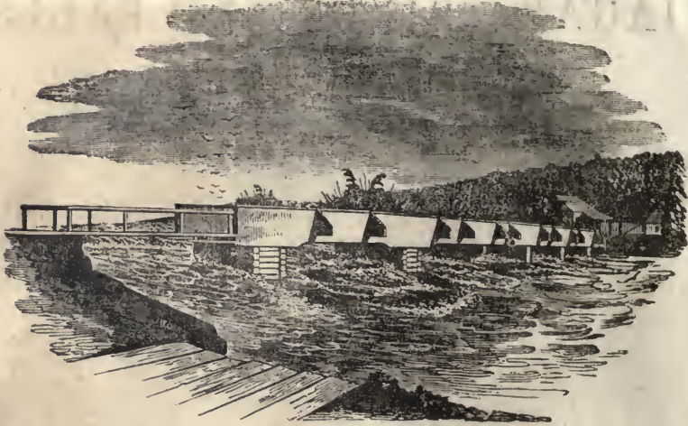
BRIDGE TO BATH ISLAND.
