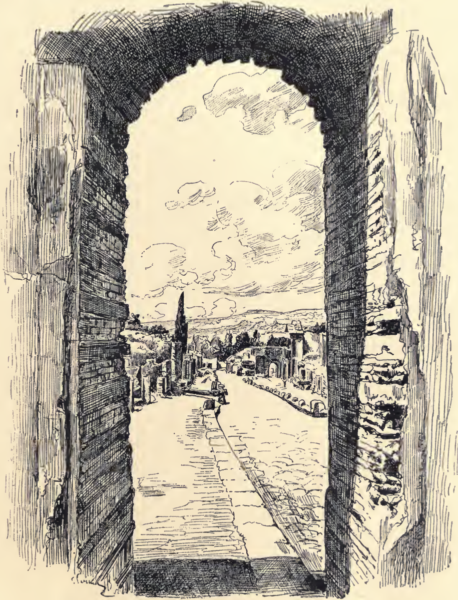
View from inside the Gate of Herculaneum
